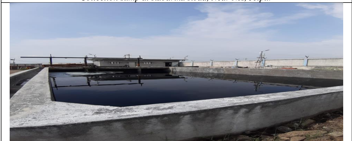
Collection sump in the premises of proposed CETP for Washing Ghat of Derdi&Monpar
