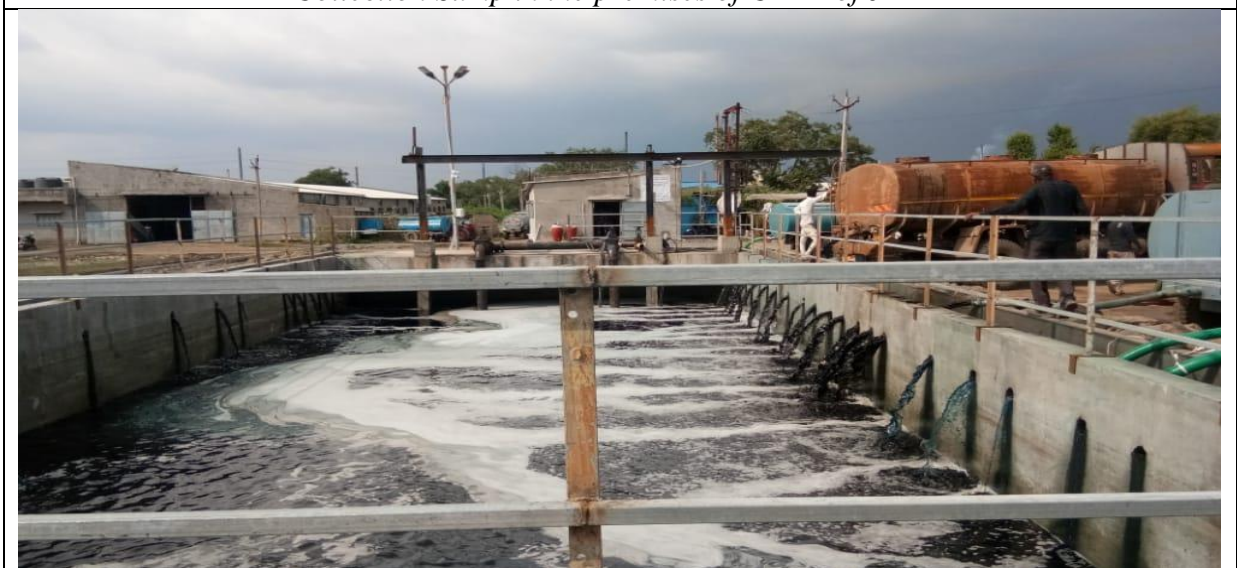
Collection sump at Rabarika Road, Near NH, Jetpur
