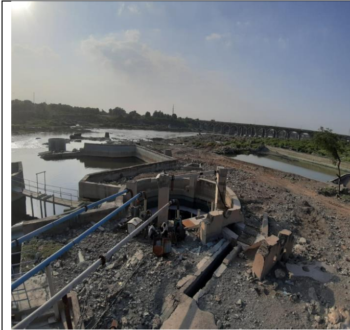
Present condition of collection sump located in river Bhadar
