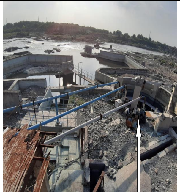
Collection well located in River bed of Bhadar & in operating condition.
