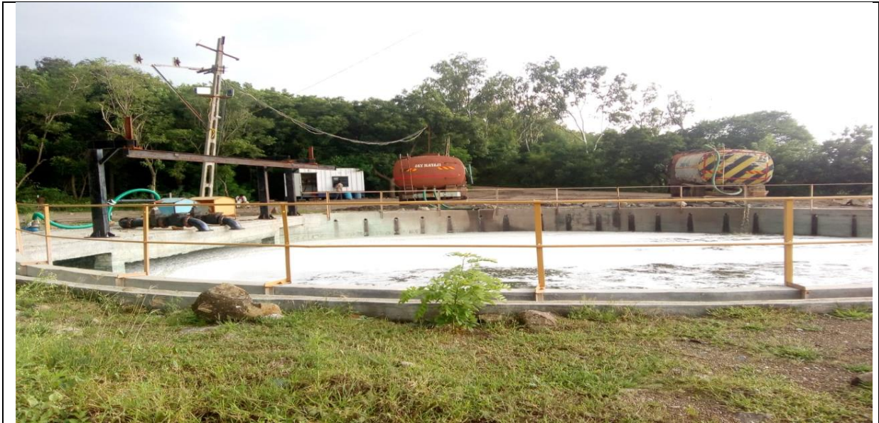
Collection Sump in the premises of CETP of JDPA
