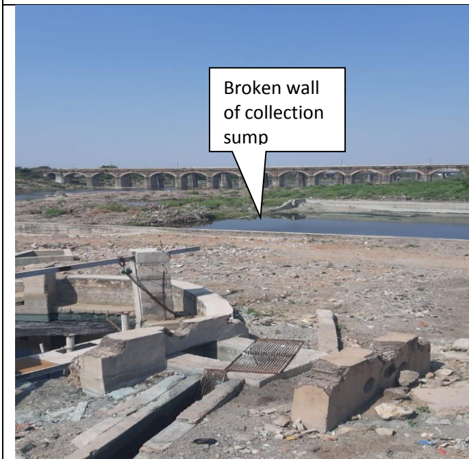
Broken wall of collection sump
